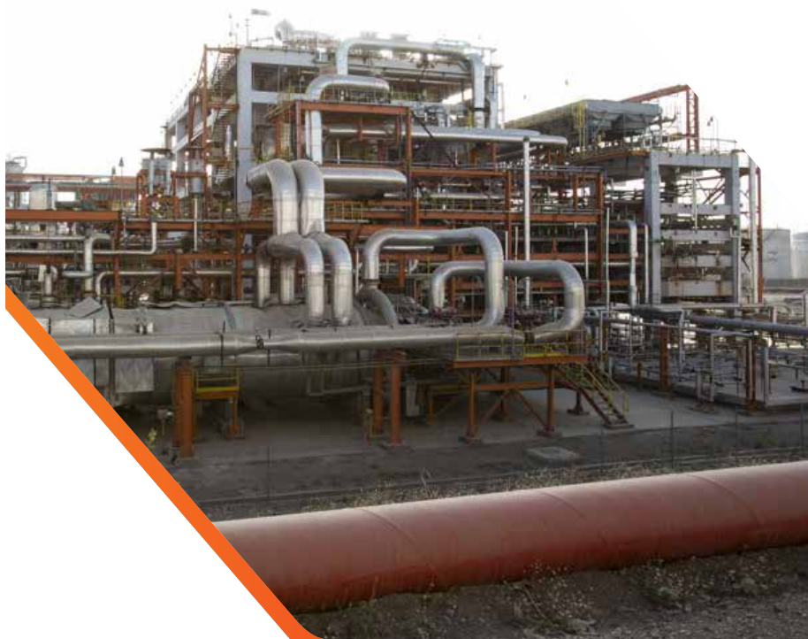
■ New Sulphur Recovery Unit at Vadinar
