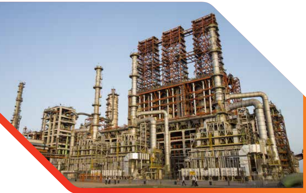
Delayed Coker Unit (DCU) at Vadinar
