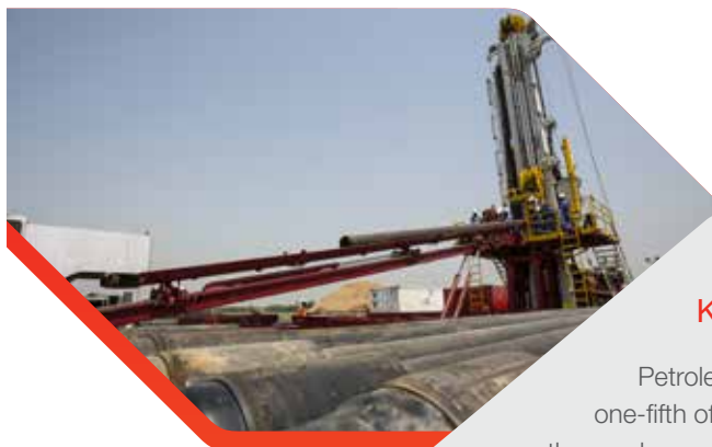
■ CBM well drilling work in progress at Raniganj
