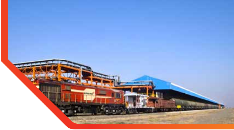
■ Rail Gantry at Vadinar
