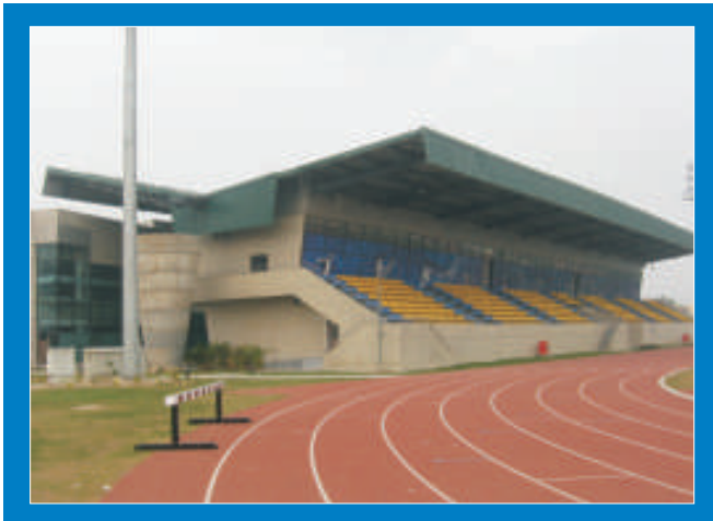
Design, Supply, Erection of Steel Structures at CWG village, Akshardham, New Delhi
