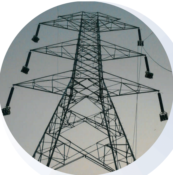
Construction of 400 KV transmission line
