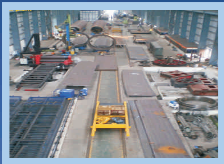
Inside view of the Plant
