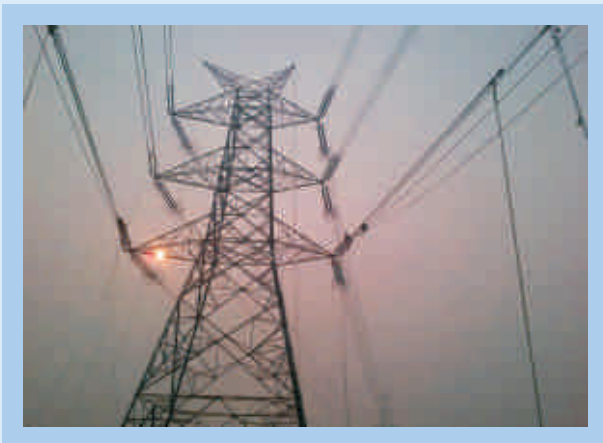
Power Transmission work for HVPNL
