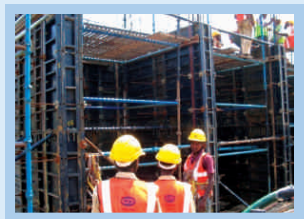
Form Work System for Lift
