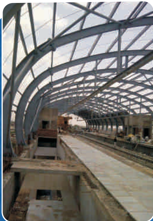
Complete steel roofing system for Jaipur Metro
