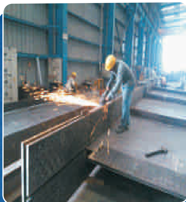
Finishing of Major Bridge Structure
