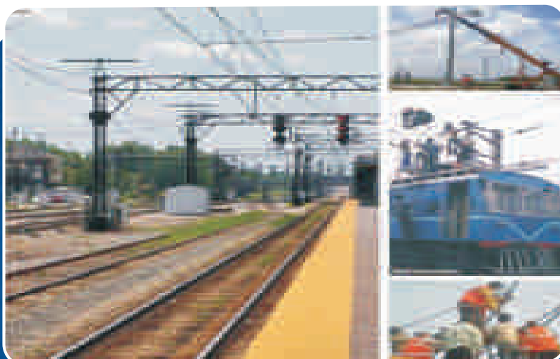
Railway Overhead Electrification
