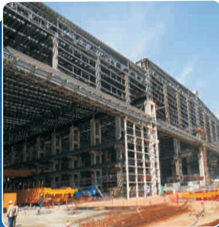
Supply & Erection of automatic shipyard door at Brazil
