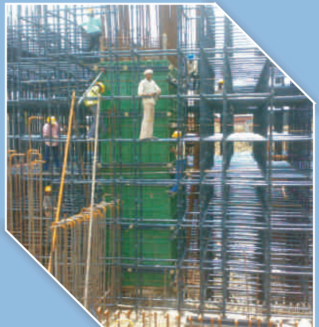
Column erection at Koradi, Nagpur
