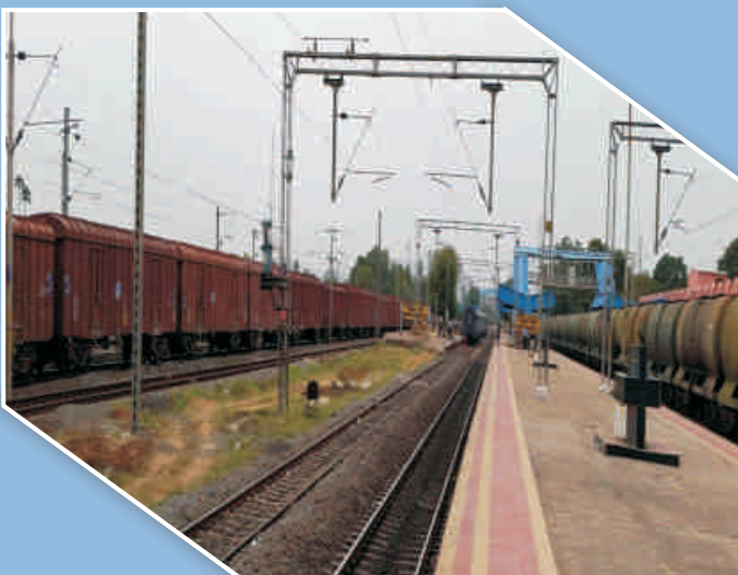
Railway Overhead Electrification
