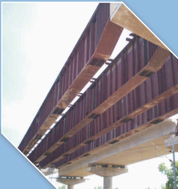
Railway over Bridge supplied for Moradabad –Bareilly Expressway
