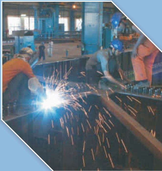
Steel Structure Fabrication works
