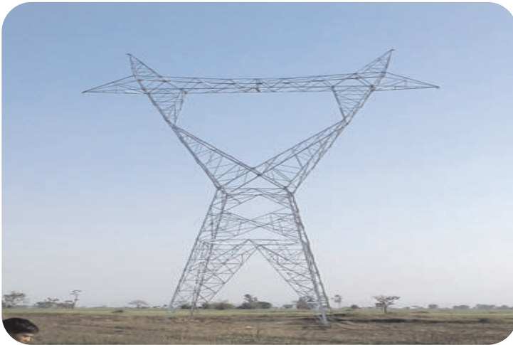
400kV Tower Erection at Allahabad
