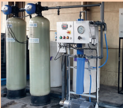
Installation of RO plant, Arockia Home for the aged, Tamil Nadu
