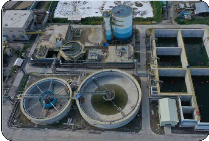
Birds eye view of complete Waste Water Treatment System for a leading paper manufacturer
