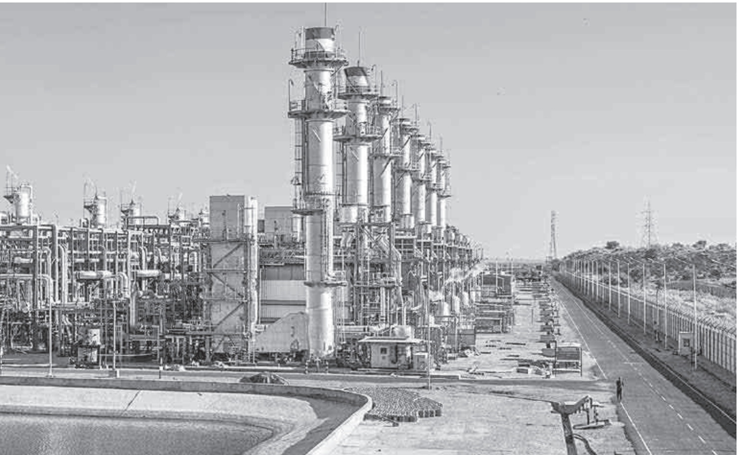
Mangala Processing Terminal, Barmer
