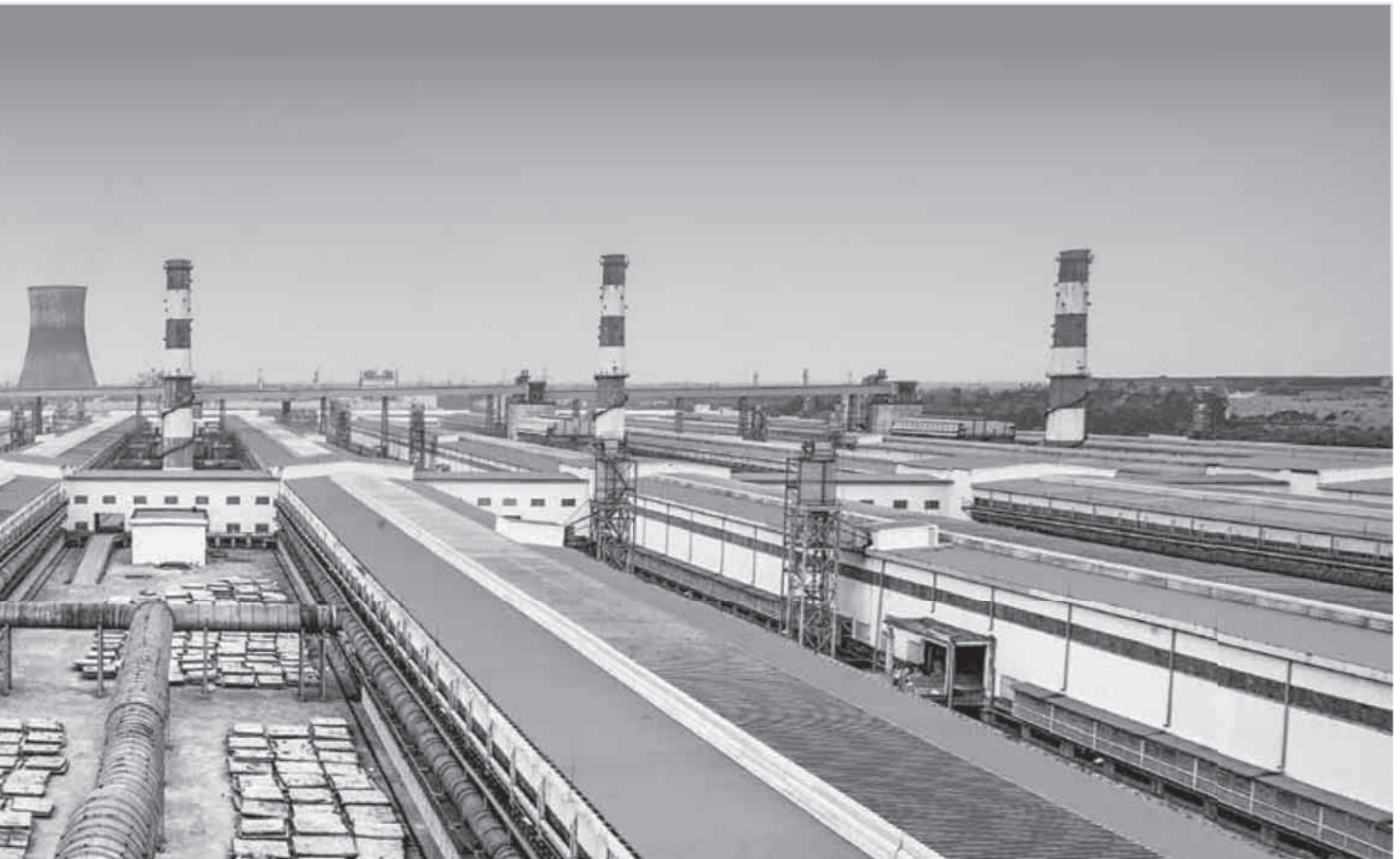
Jharsuguda smelter and power operations
