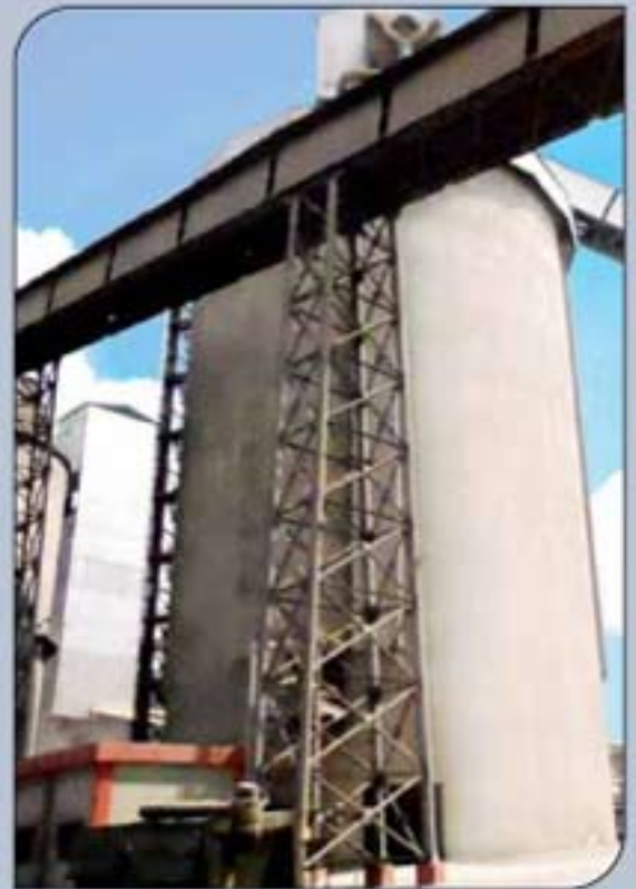
The new clinker silo at Satna Cement Works, Madhya Pradesh
