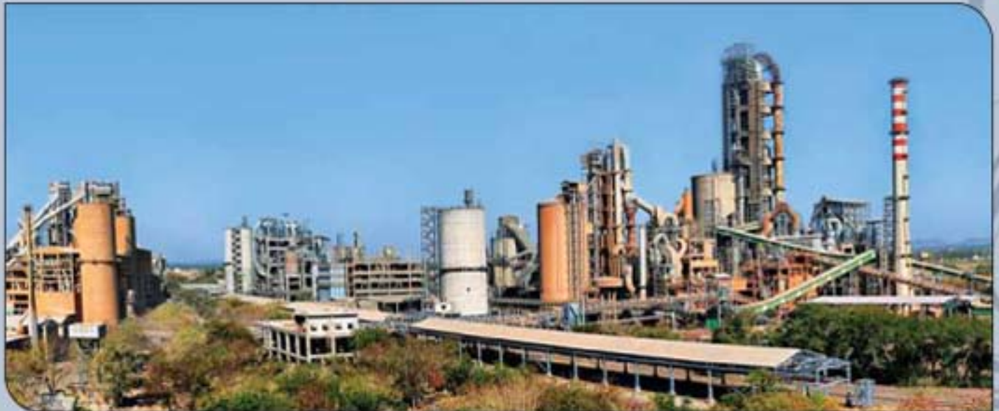
A panoramic view of Birla Cement Works, Chanderia Cement Works and New Chanderia Cement Works at Rajasthan
