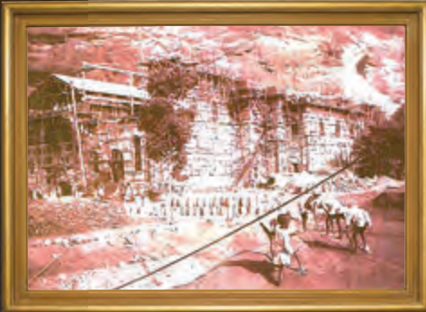
Construction at Khopoli Power House
