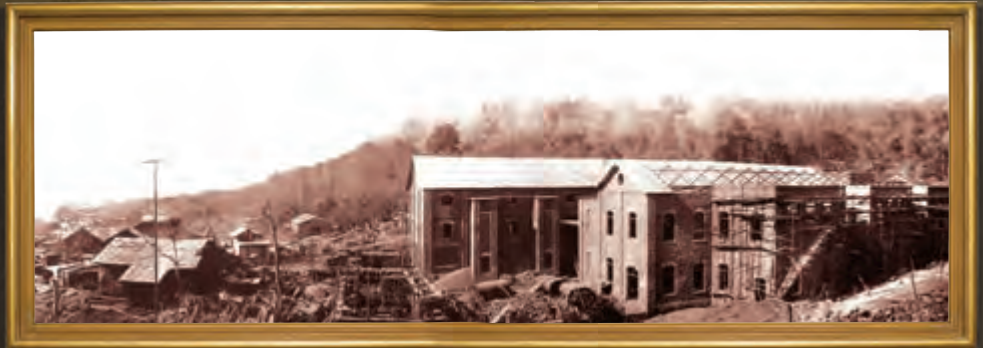
Old Power House under construction
