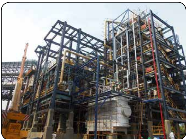
PA Plant Revamp : Oxidation Section - Ranipet
