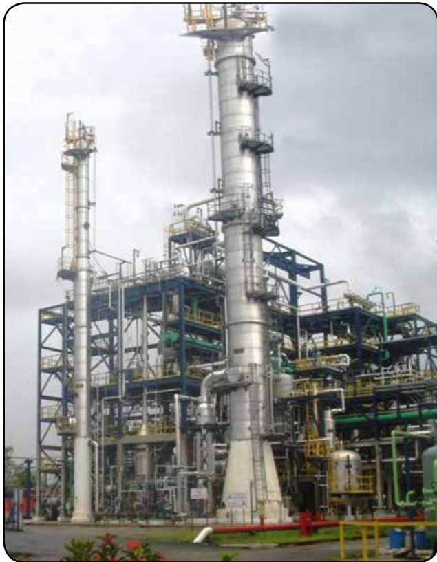
Butane Processing and Butamer Plant: Malaysia
