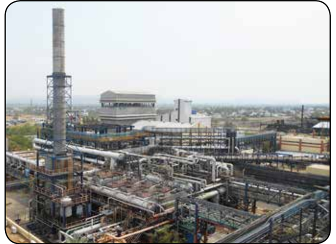
PA Plant - Ranipet, during revamp
