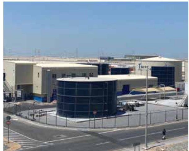
||||| NFPC Effluent Treatment Plant, Abu Dhabi
