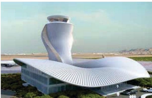
|||||| Fujairah International Airport Expansion, Fujairah, UAE
