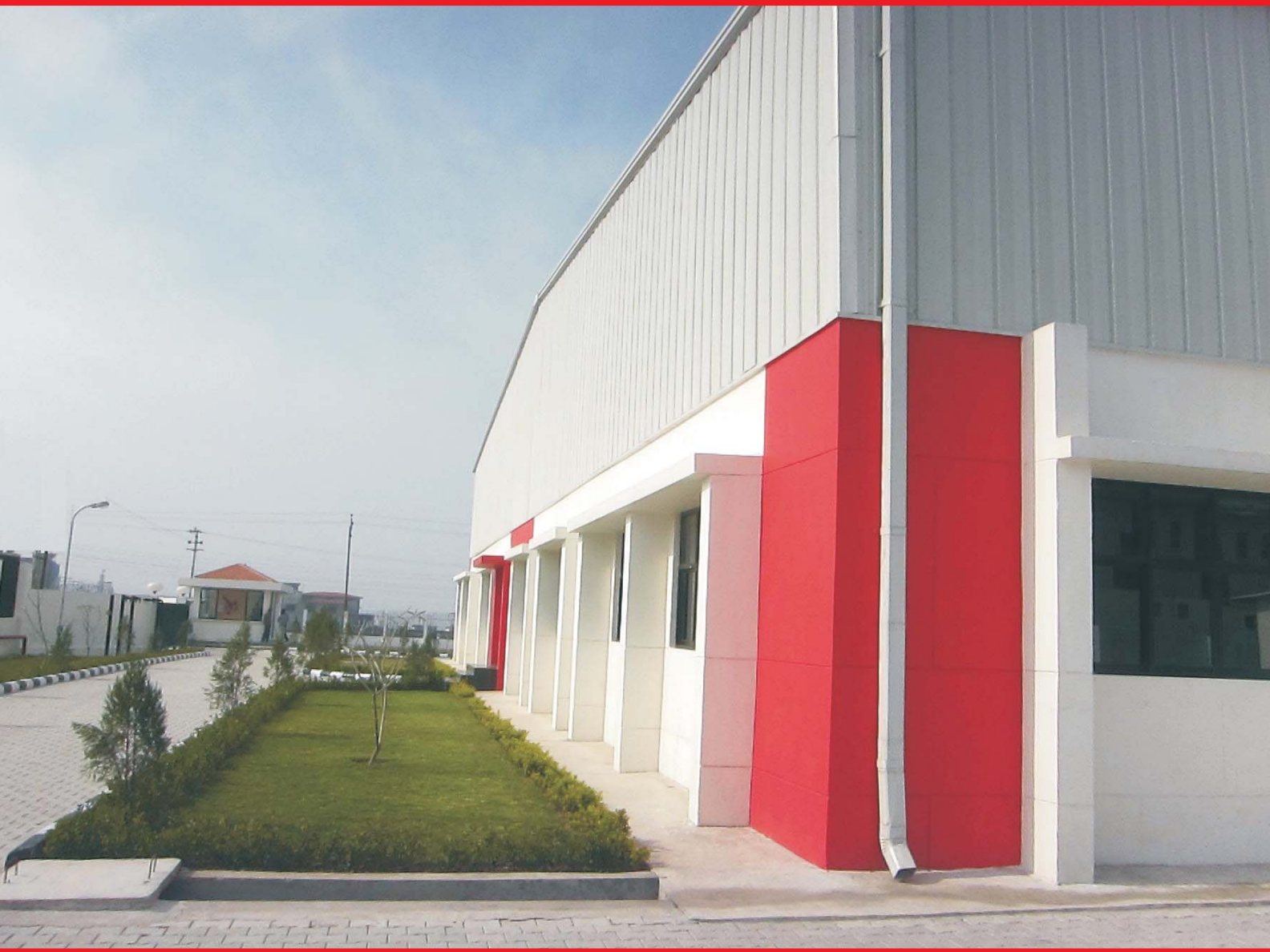
New Uttarakhand Plant
