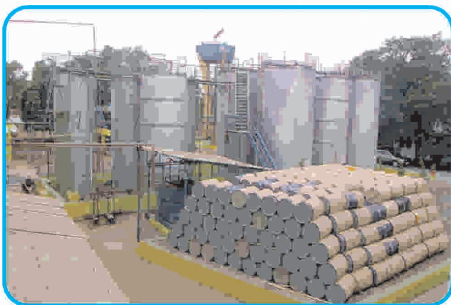
Raw Material Storage Facility
