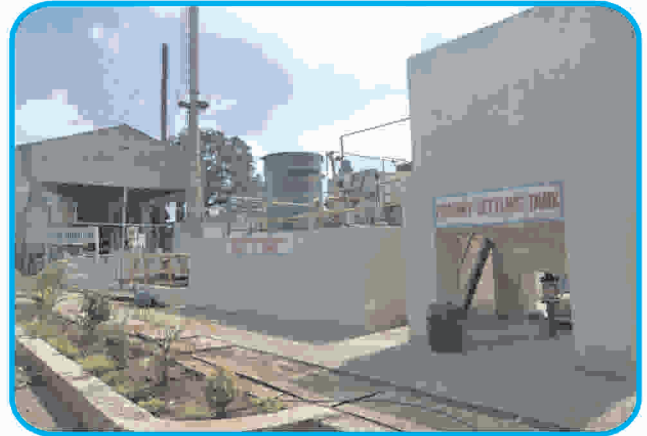
New Effluent Treatment Plant
