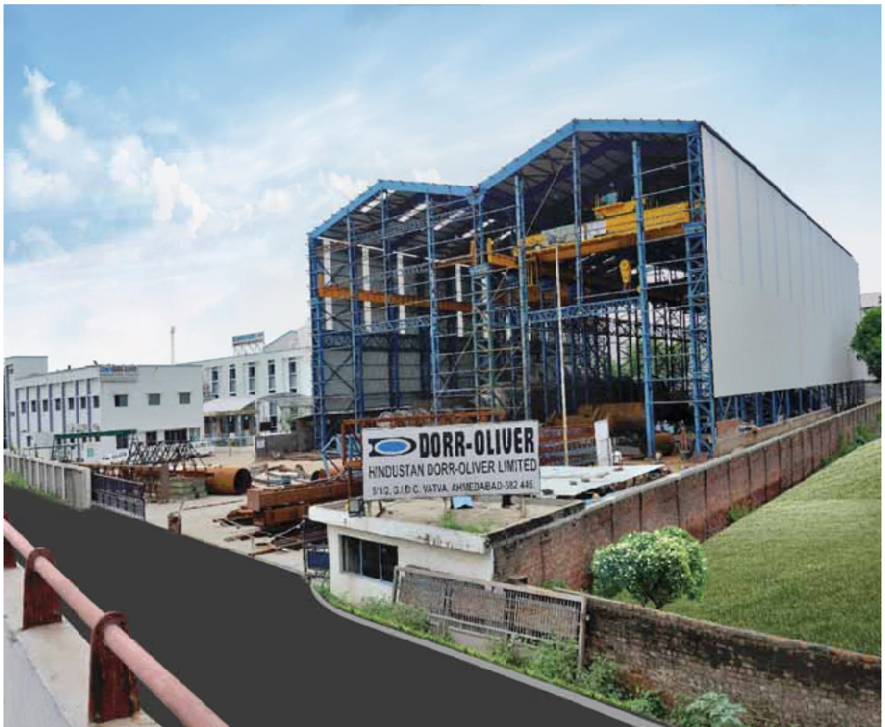
NEW FABRICATION FACILITY - BAY 5 AND 6
