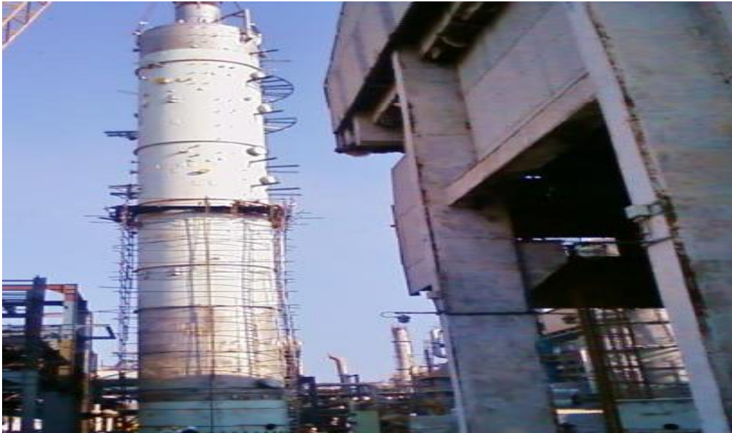
CO2 Absorber supplied to Tecnimont weighing 120 mt.
