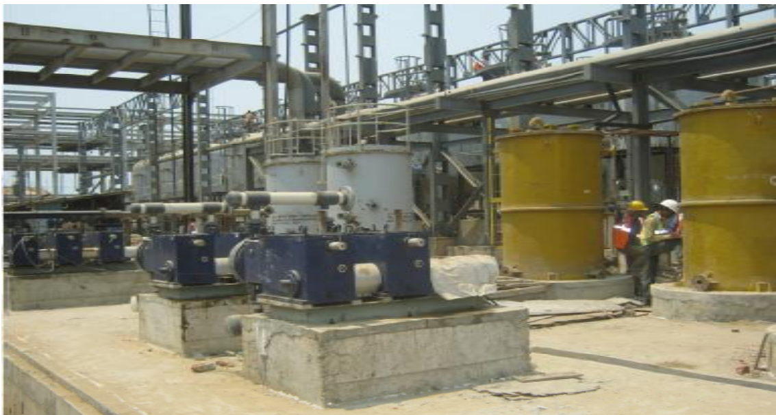
LSTK – Dimineralised Water and Condensate Polishing Unit for Indian Oil Corporation Ltd., Paradip, Odisha.
