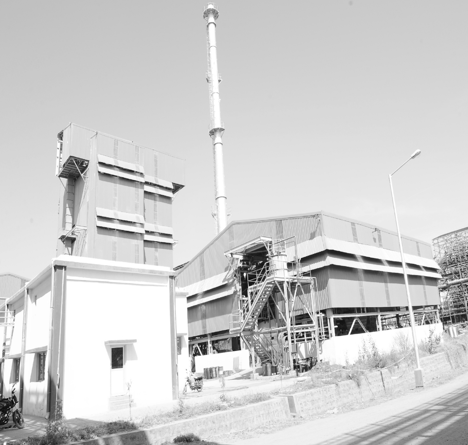
Steam Generation System- UCIL
