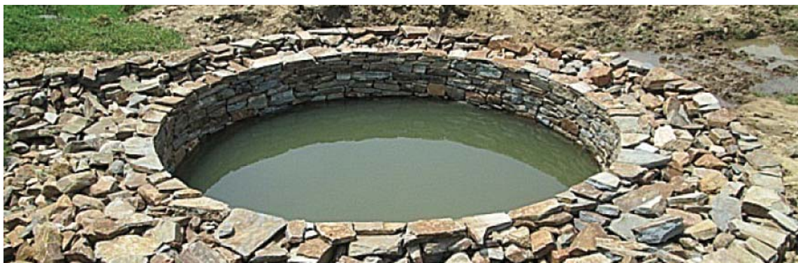
Well Renovation in Progress at Patratu in Ramgarh
