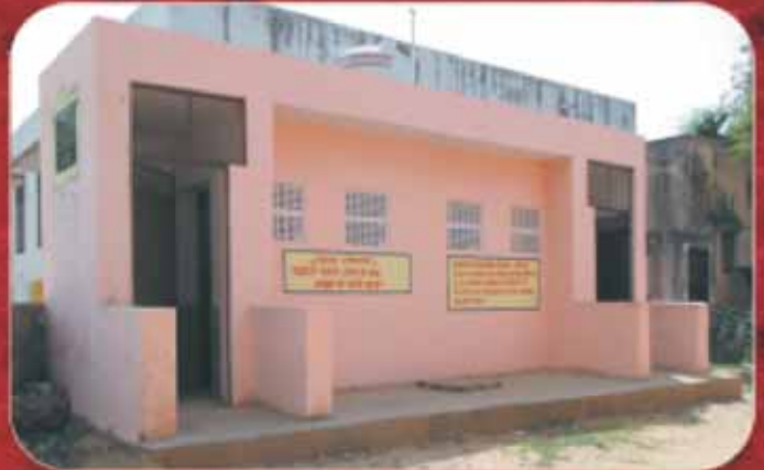
Constructed new toilet( Apni Azadi) at Girls Upper primary school Dhodsar
