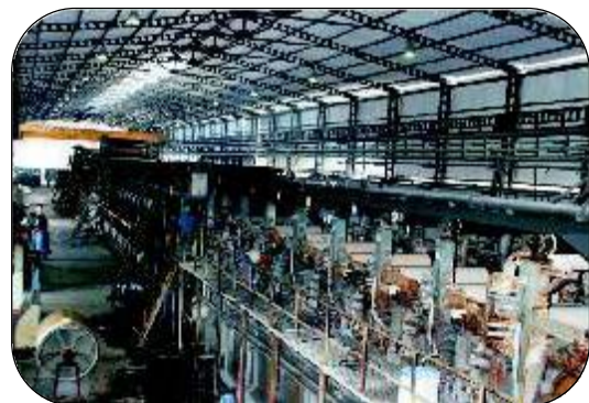
Second Machine under Installation - at Glance
