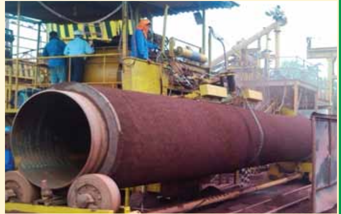
“Concrete Weight coating” for Offshore Pipeline in progress
