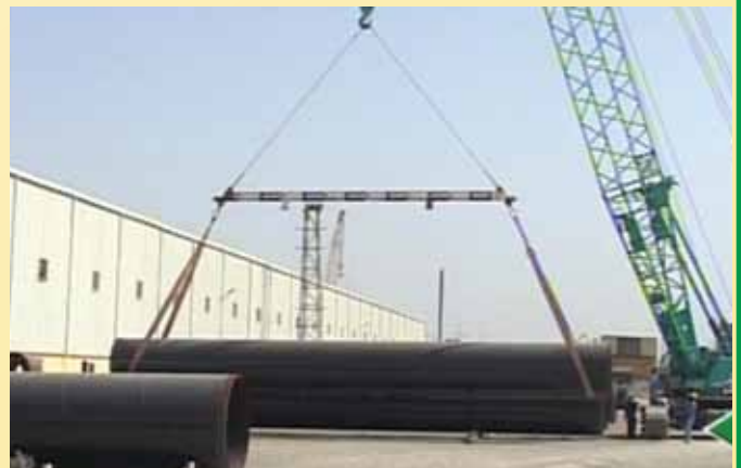
SECURE Pipe Handling at PSL’s Pipe Yard
