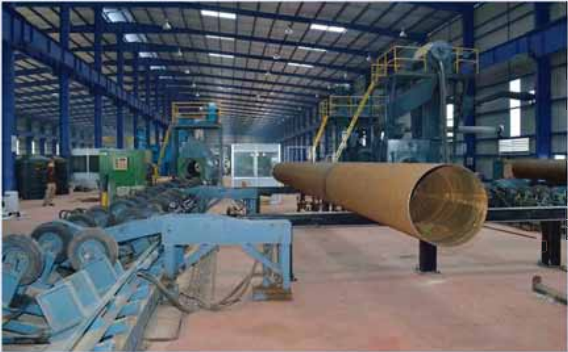
Views of 3LPE/FBE Coating plant established at PSL - Jaipur
