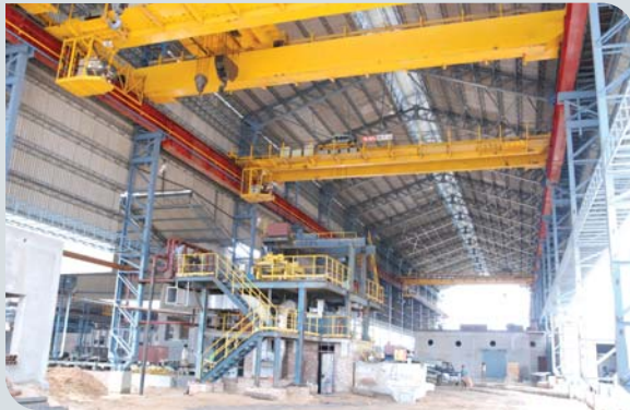
STEEL MELTING SHOP SHED
