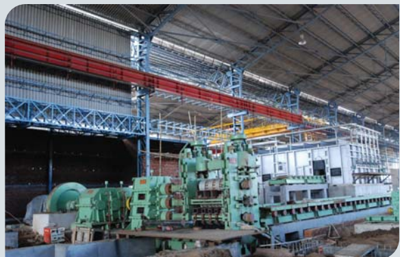
ROUGHING MILL AREA
