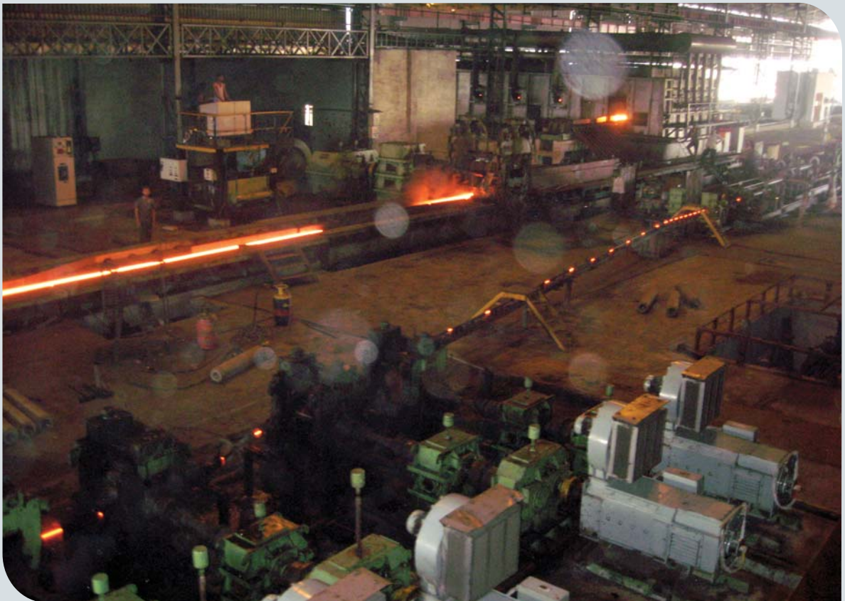
A VIEW OF TMT ROLLING MILL
