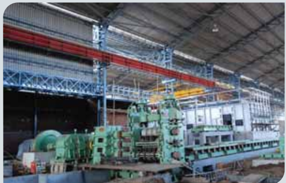
ROUGHING MILL AREA
