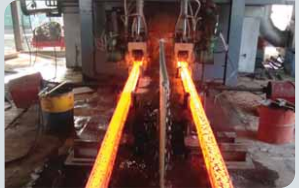
Continuous Casting Plant at Bihta
