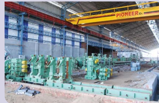
ROLLING MILL AREA
