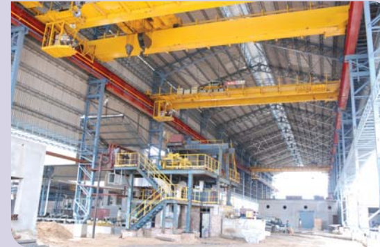
STEEL MELTING SHOP SHED
