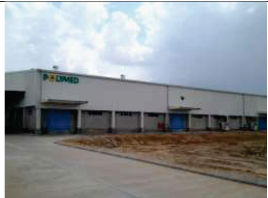
Unit IV at SEZ Jaipur, Rajasthan (New Facility)
