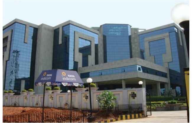
BUILDING HOUSING ACCENTIA'S UNIT I, BHUBANESWAR
