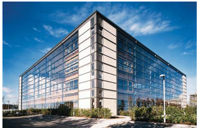
BUILDING HOUSING ACCENTIA'S OFFICE, LONDON
