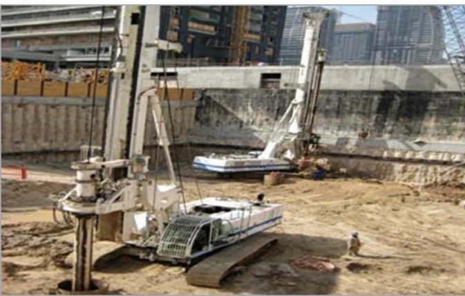
▲ Bored Pile Installation at Dubai.
