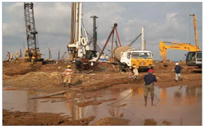
▲ Concreting work at IOCL Refinery Paradip, Orissa.
