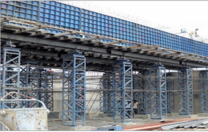
▲ Lebad-Manpur Section (SH-31) BOT Road
