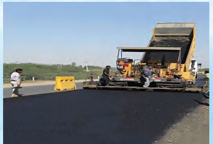
BC laying in progress - Bhuj Bhachau-Kachchh
