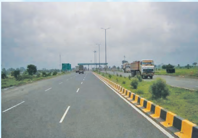
Lebad - Manpur 'BOT Project'
