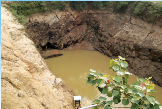
Dewatering at Banaso Konar Tunnel Project, Hazaribagh, Jharkhand
