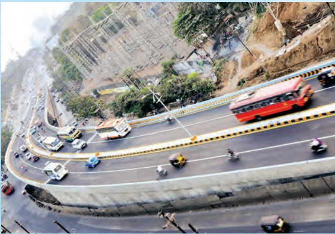
Ghodbundar Flyover at Patlipada, Thane
