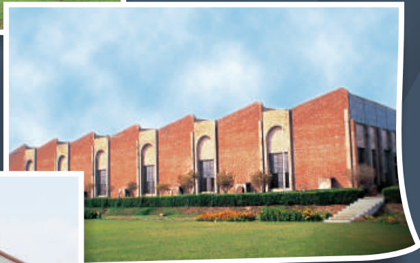
Switchgear Plant, Murthal
