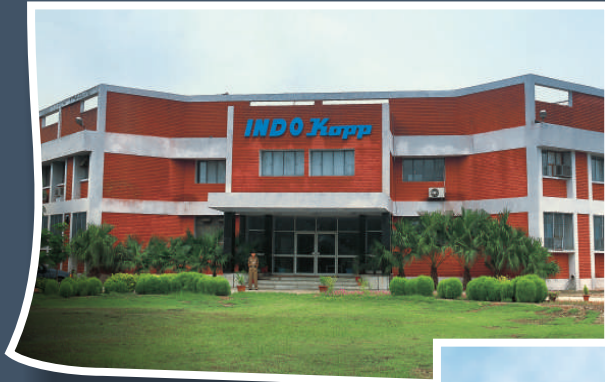
Switchgear Plant, Noida
