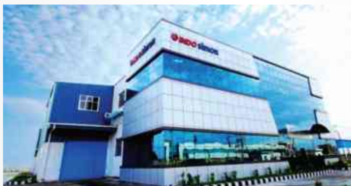
Modular Switches Plant Haridwar
