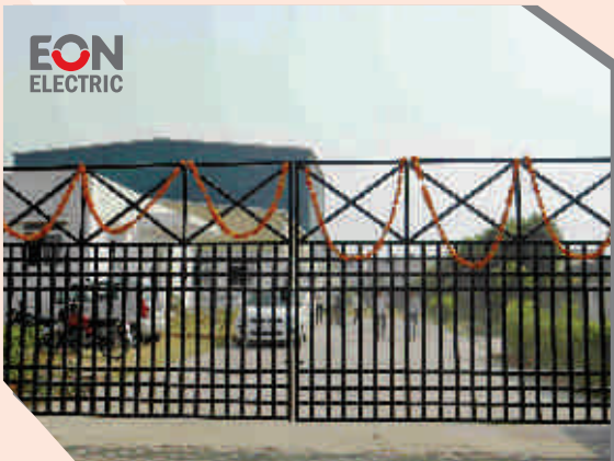
Fans & LED Bulb Plant at Haridwar
