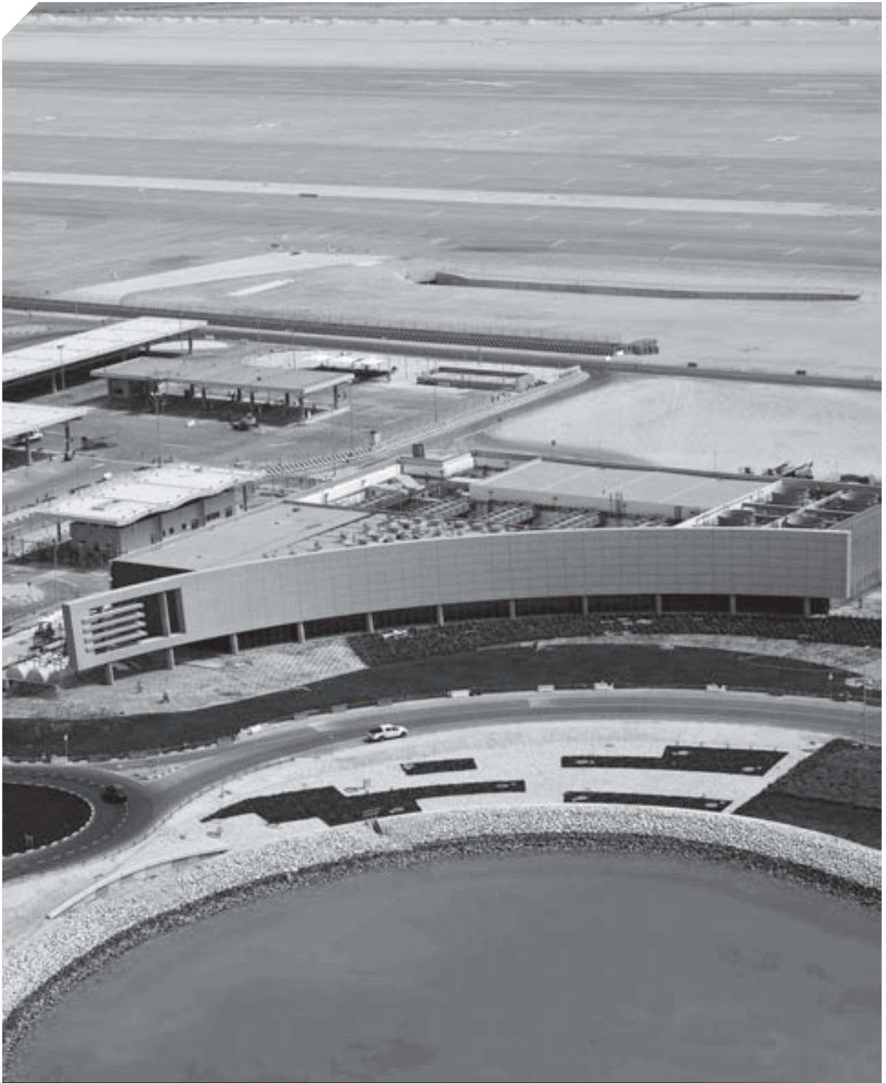
FUEL SYSTEMS FOR NEW DOHA INTERNATIONAL AIRPORT, QATAR
