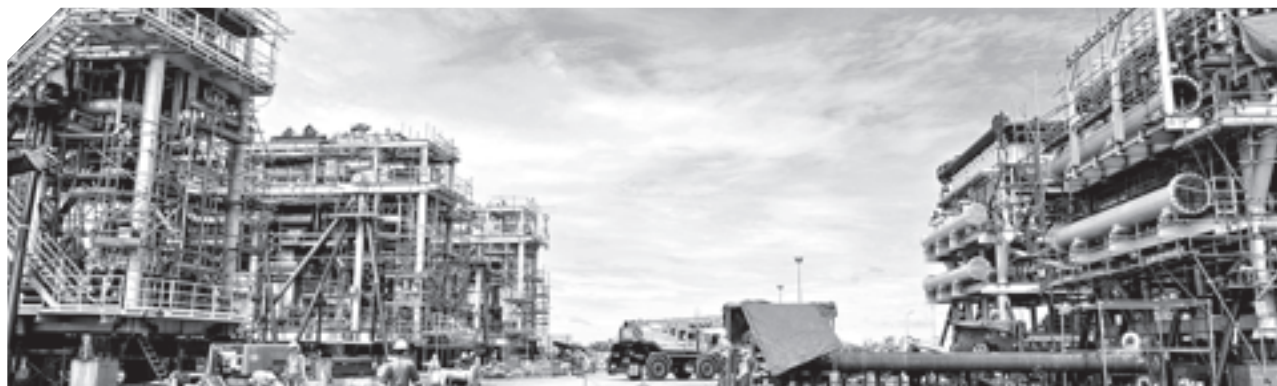
ASSEMBLED MODULE FOR LOAD-OUT ONTO BARGE, PCF PROJECT, THAILAND
