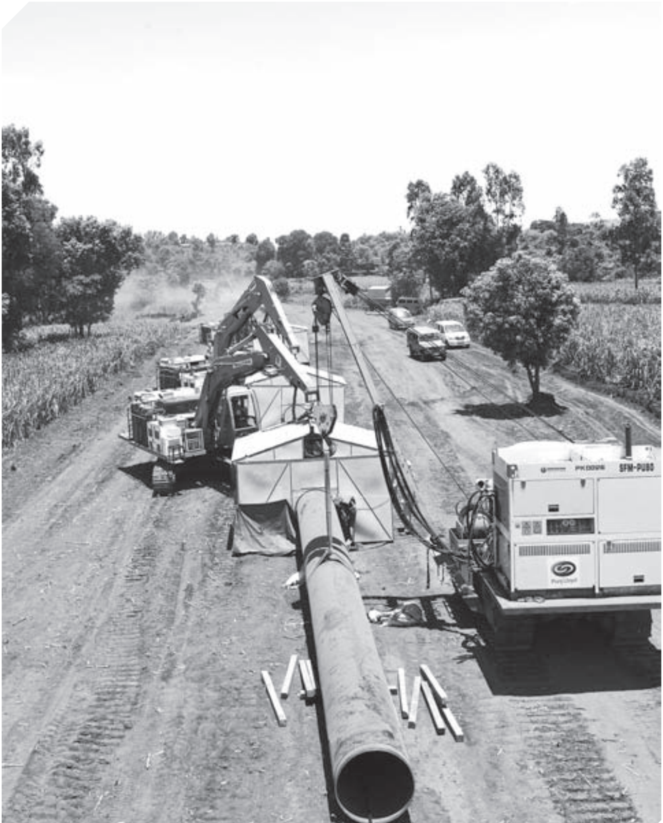
AUTOMATIC WELDING MACHINES DEPLOYED AT THE DABHOL BANGALORE PIPELINE, INDIA
