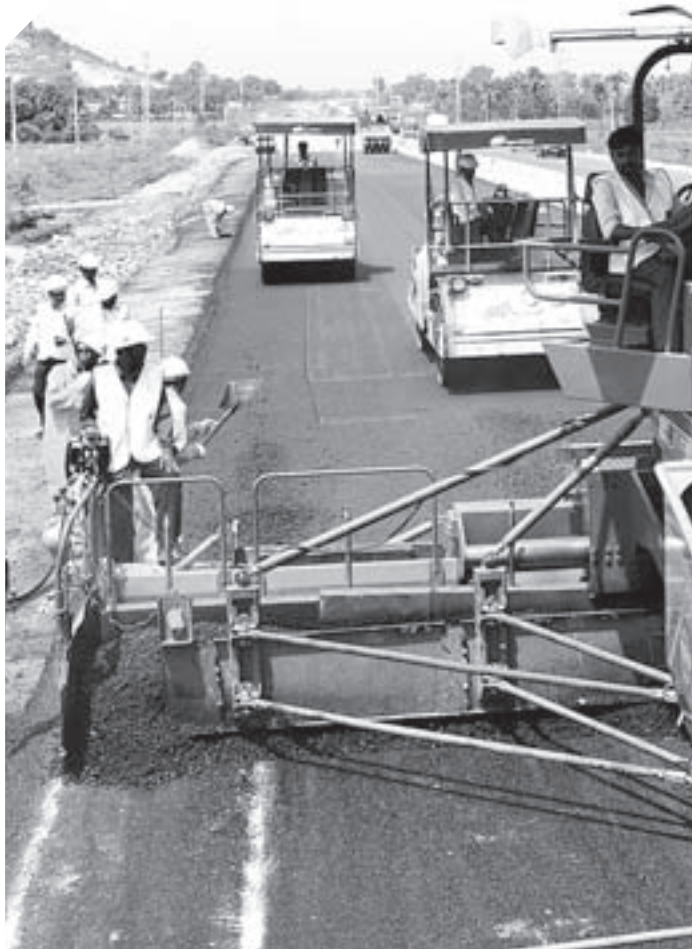
HYDERABAD VIJAYAWADA ROAD PROJECT, INDIA
