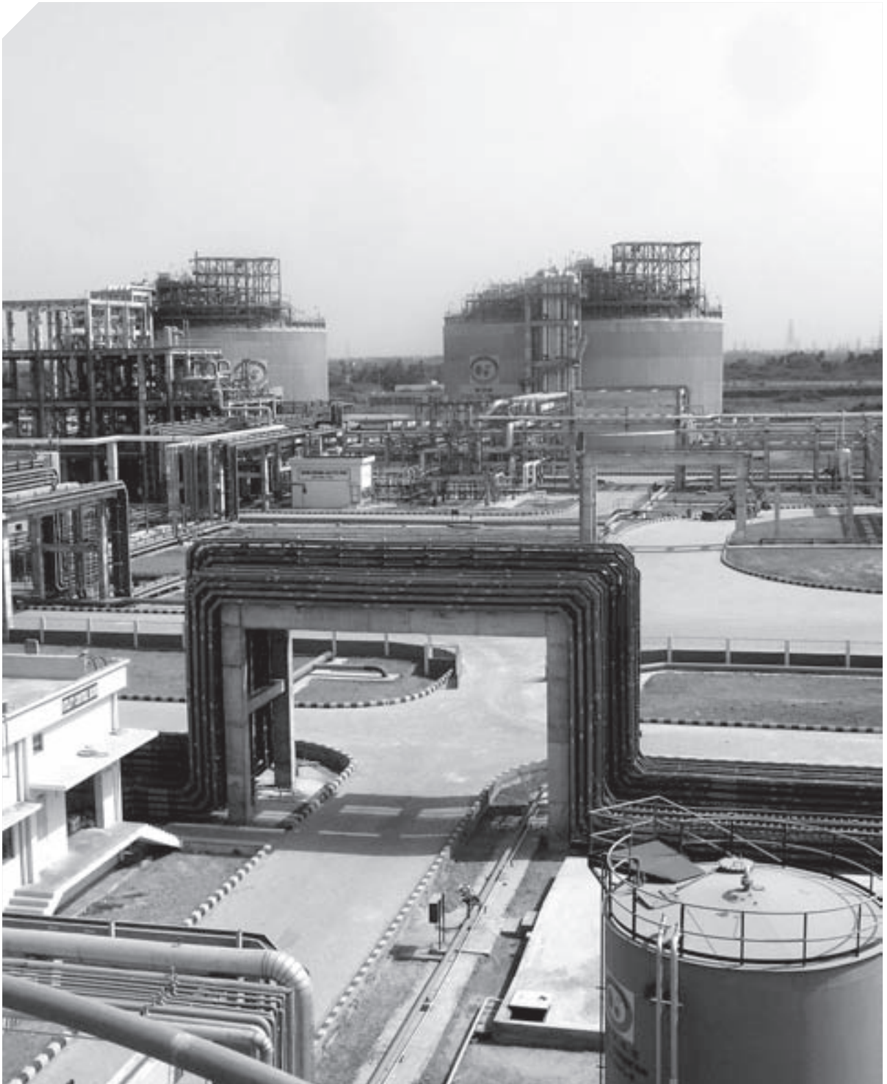
LPG/PROPANE/BUTANE IMPORT TERMINAL, ENNORE, TAMIL NADU, INDIA
