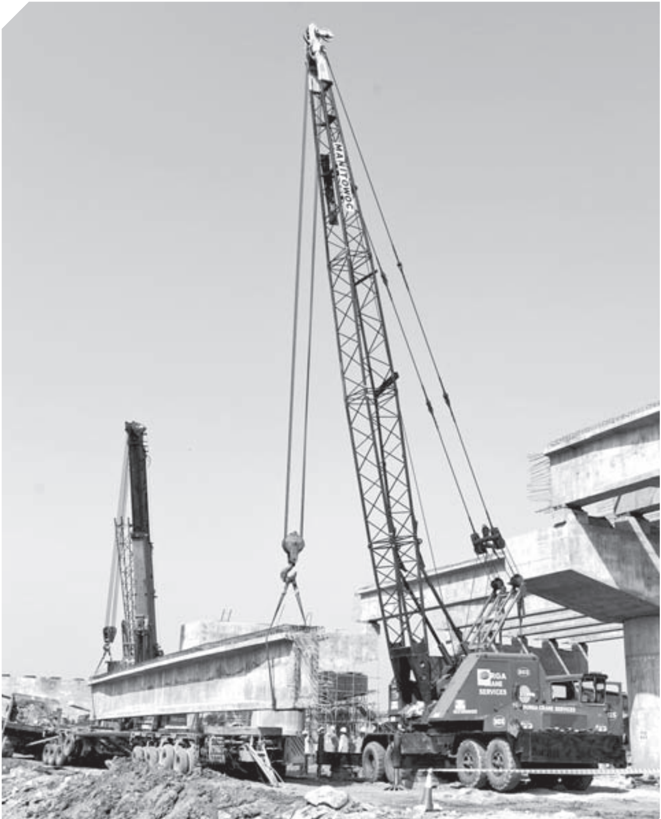
GRADE SEPARATOR BEING CONSTRUCTED ON HYDERABAD VIJAYAWADA HIGHWAY PROJECT, INDIA
