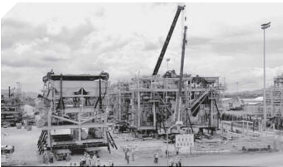
ASSEMBLED MODULES FOR PLATFORM COMPRESSION FACILITIES (PCF) PROJECT, THAILAND
