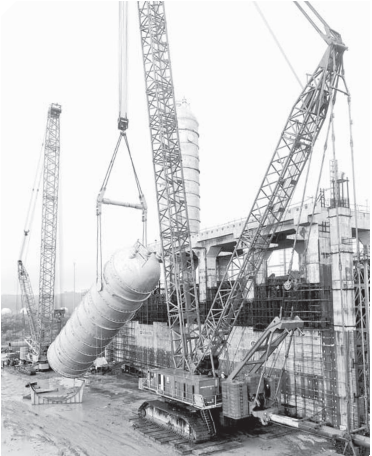
HEAVY LIFTING OF COKE DRUM AT MANGALORE REFINERY, INDIA
