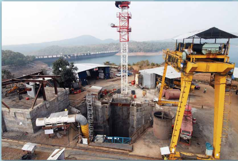
Opening Shaft (Modak Sagar Tunnel Project)
