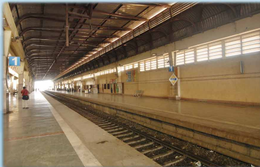
Completed Railway Station Project At Navi Mumbai
