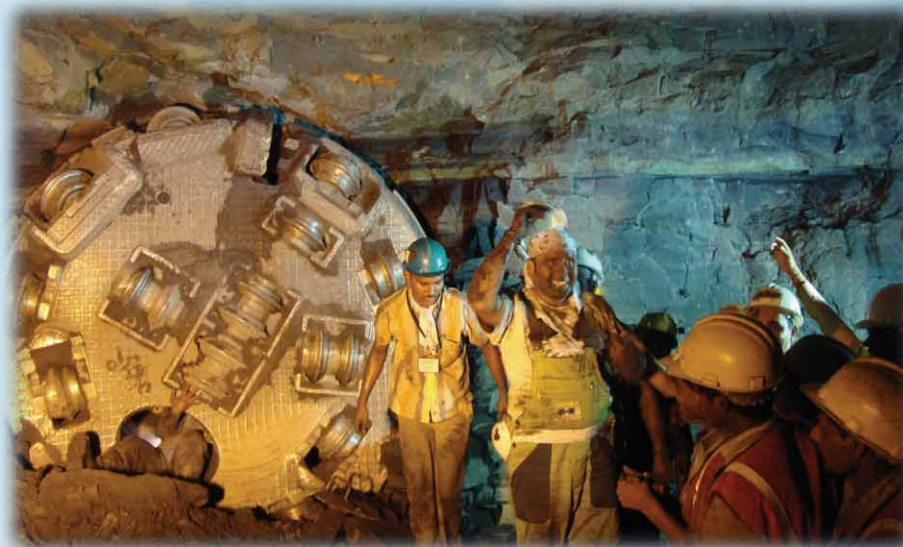
Breakthrough of Tunnel (Malabar Hill Tunnel Project Phase II)
