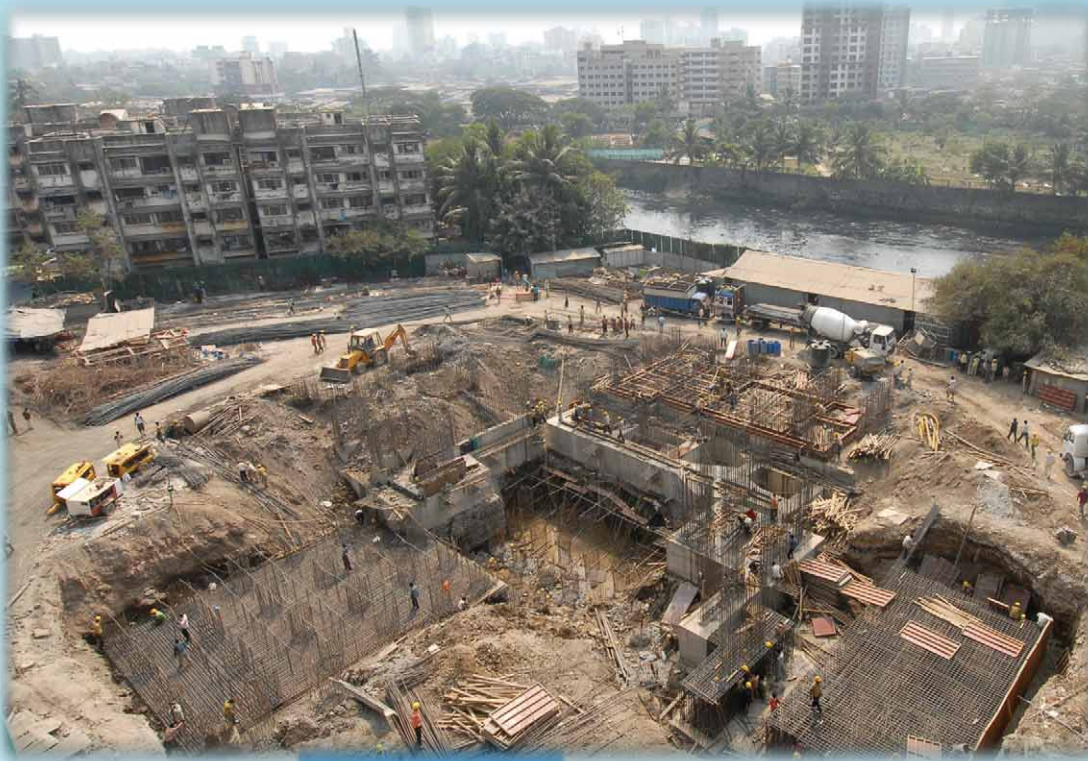
Building Construction Site
