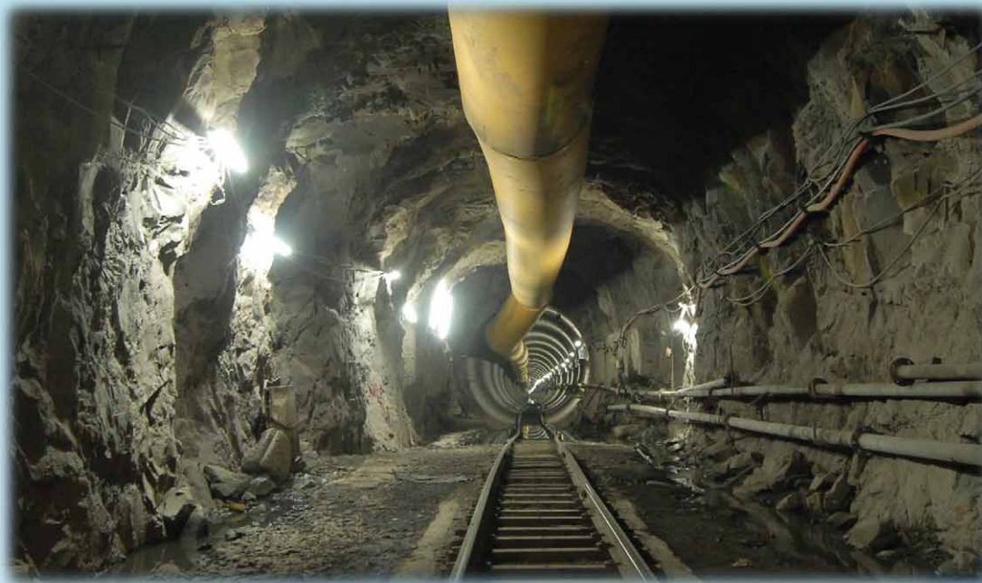
Inside View of Malabar Hill Tunnel Project
