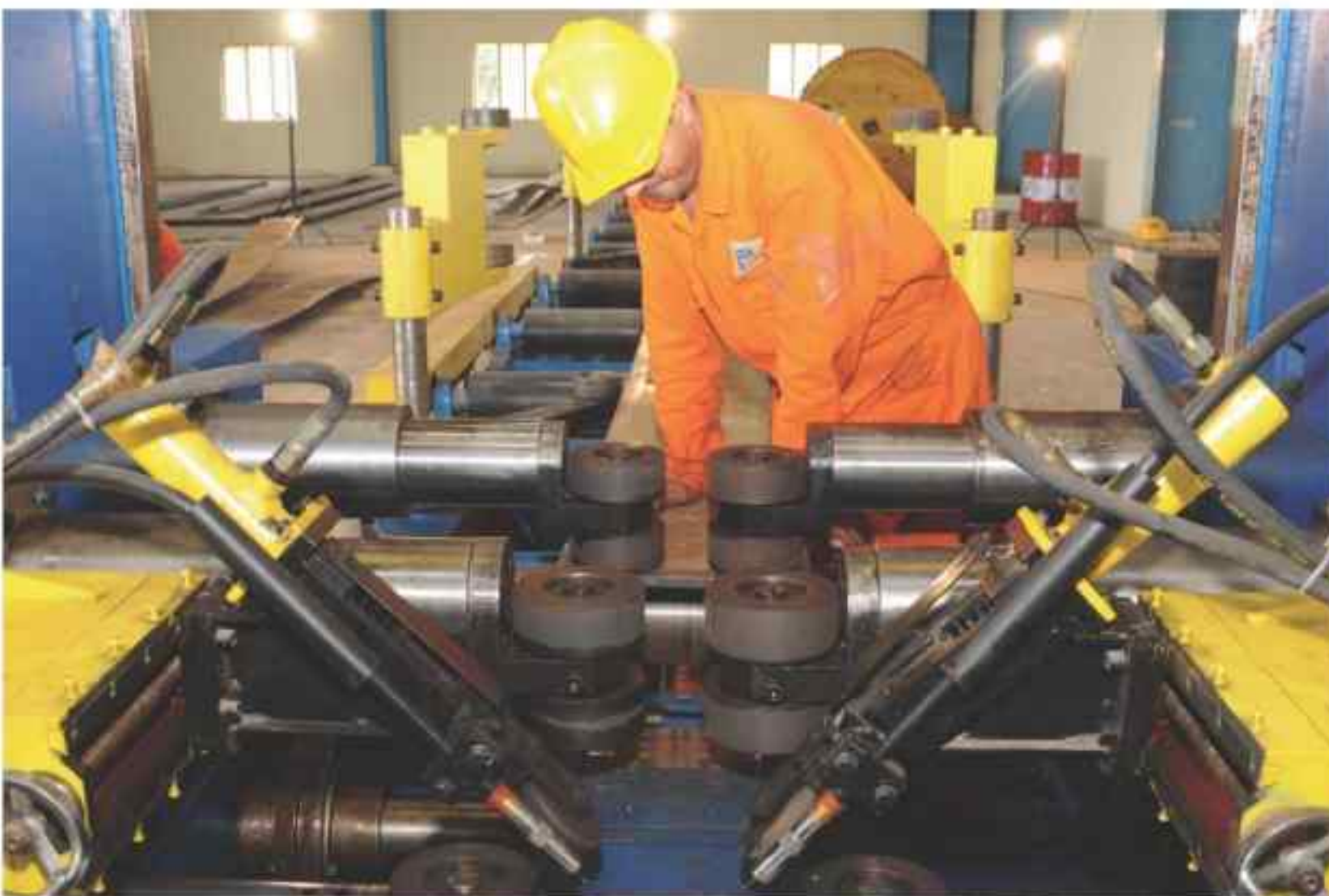
A worker at our plant at Wada
