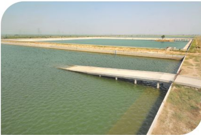
Water Supply Project – HUDA
