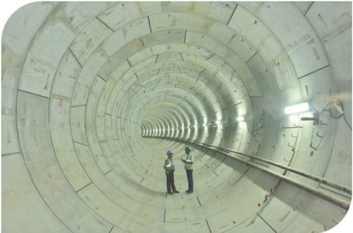
DMRC Tunnel - New Delhi
