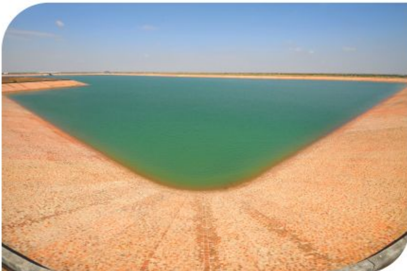
Water Supply Project - Nagaur - Rajasthan
