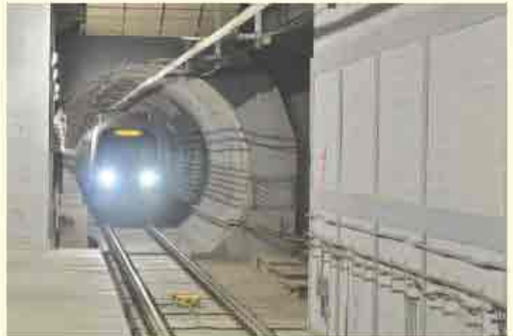
DMRC Mandi House Underground Metro Station
