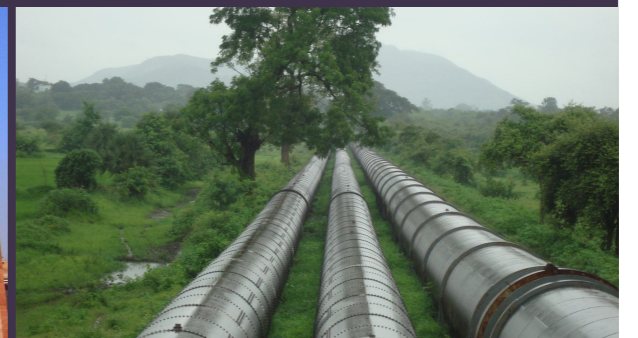
Replacement of Tansa Mains - Thane District
