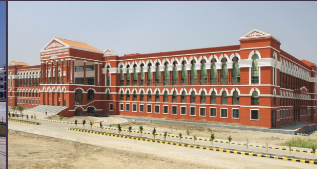
High Court Circuit Bench Building - Gulbarga, Karnataka
