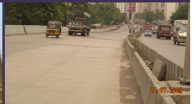
Strengthening of Jogeshwari - Vikhroli Link Road, Mumbai
