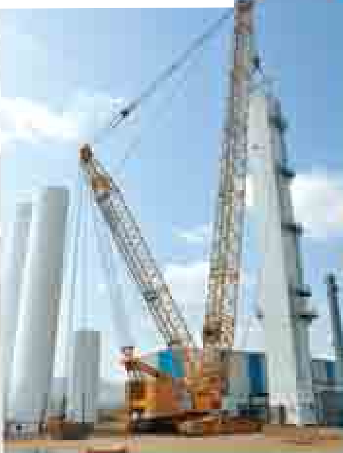
Lifting Project and Mangaon, Raigad
