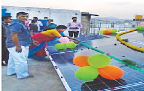
10 KVA Solar Power System
