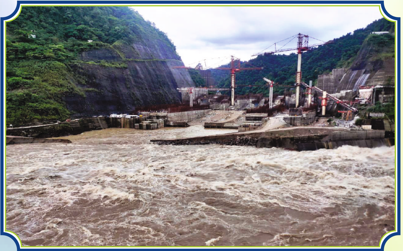
2000 MW Subansiri Lower Project (Arunachal Pradesh/ Assam) - Dam under construction
