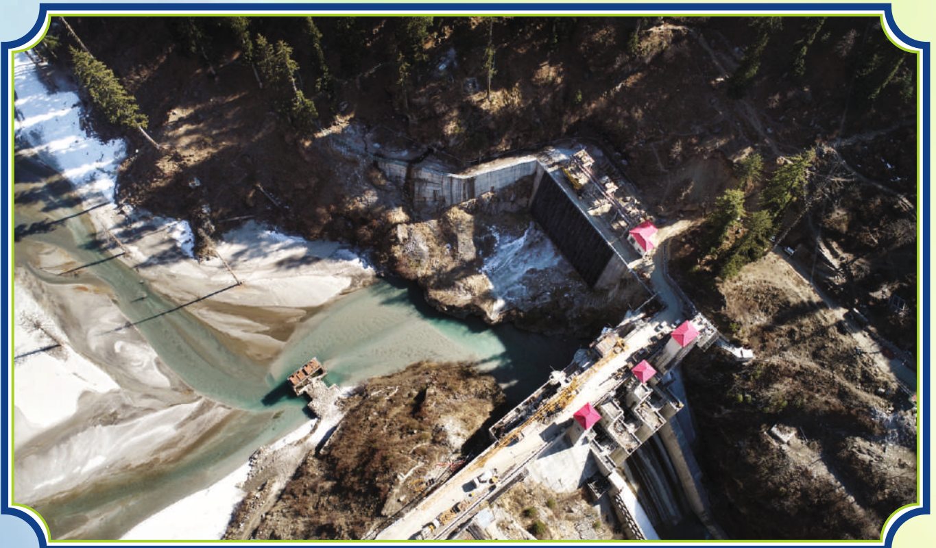
800 MW Parbati-II Project (Himachal Pradesh) - Aerial view of Dam site
