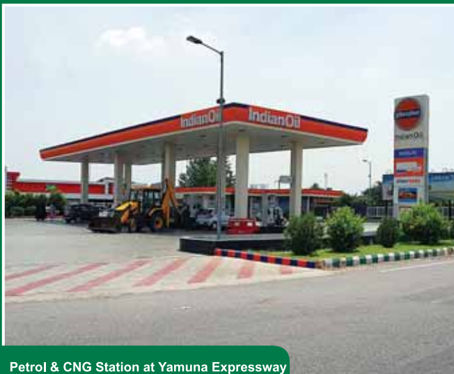
Petrol & CNG Station at Yamuna Expressway
