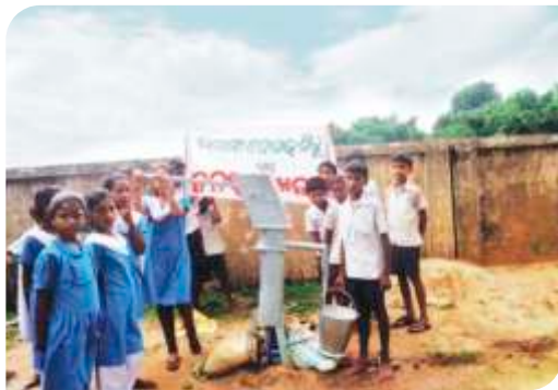
Installation of Tubewell
