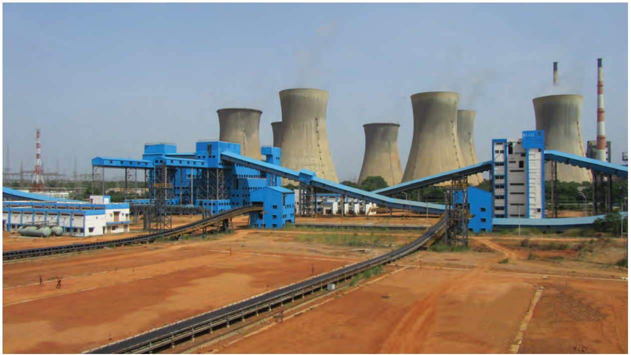
Lignite Handling System at Neyveli Lignite Corporation Limited, Neyveli for its 2X250 MW Thermal Power Plant.
