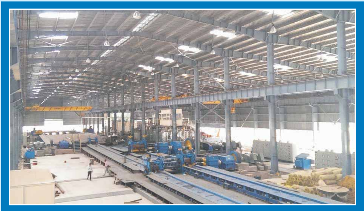
Interior view of the Steel Rolling Mill of the Company at Alwar, Rajasthan.
