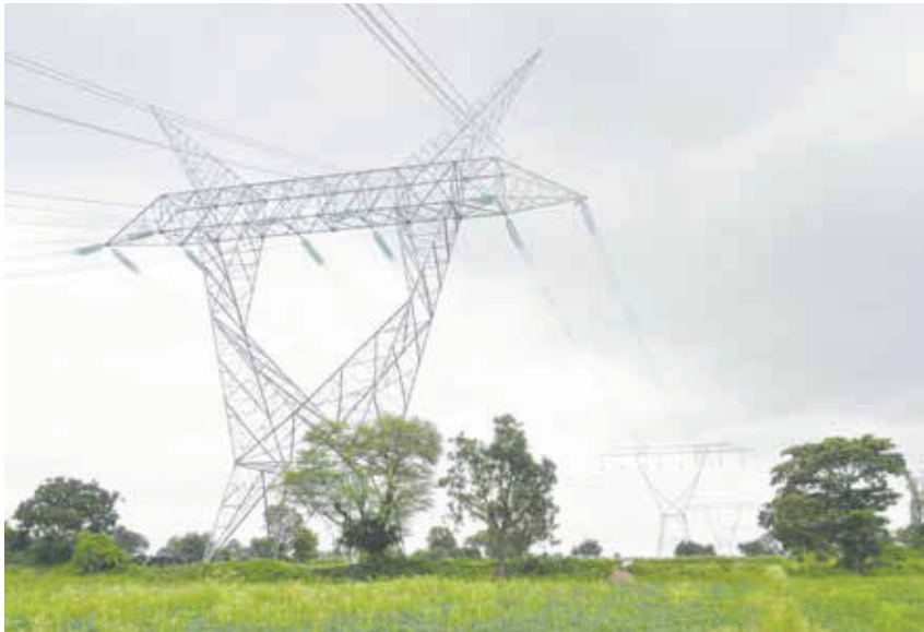
▶ 1200 kv transmission line tower under execution in Wardha, Maharashtra
