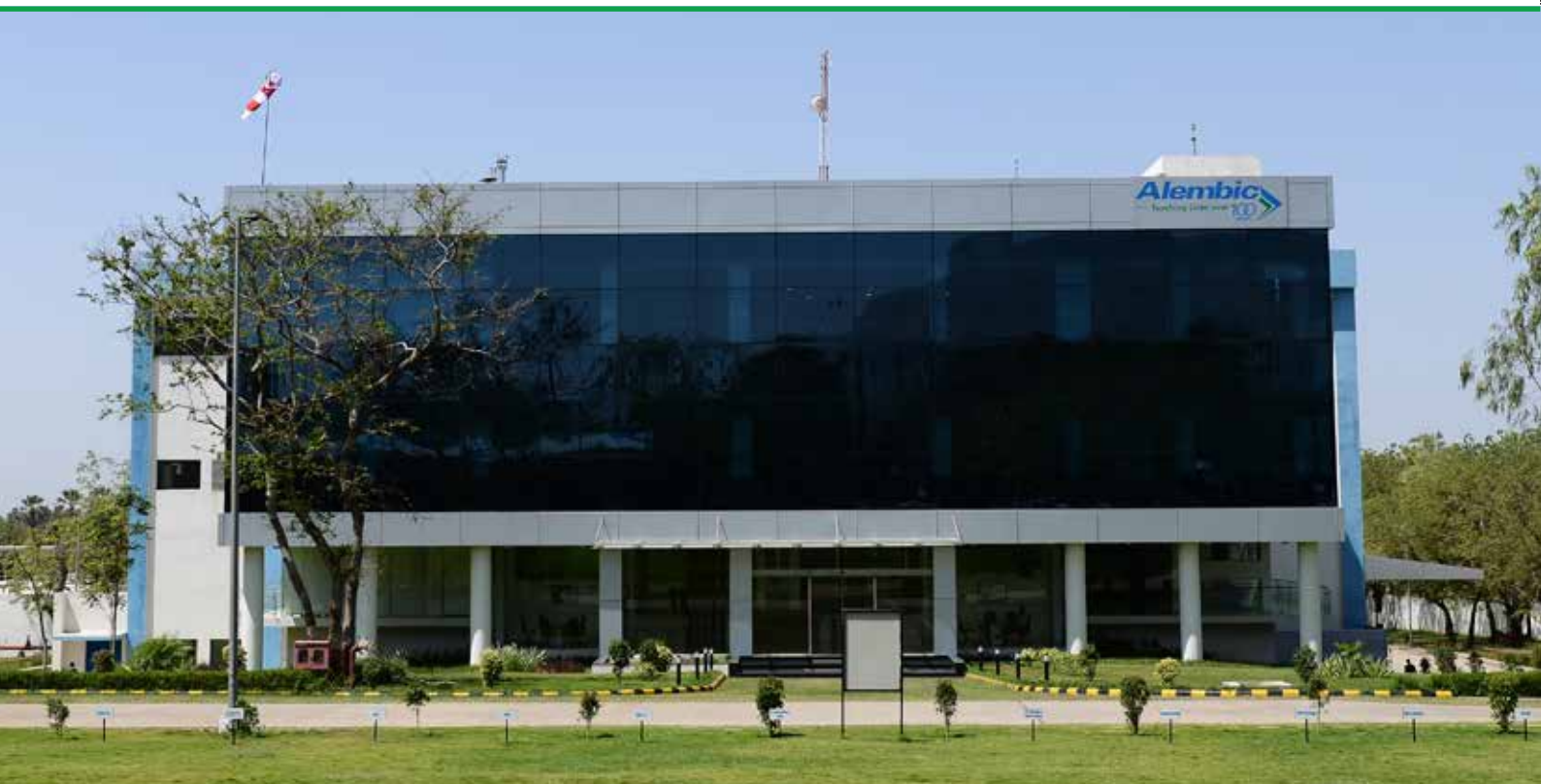
Oncology injectable and OSD plant (F2), Panelav
