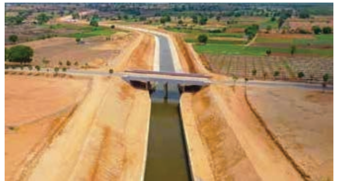
Ramayampet Canal Works, Siddipet, Telangana
