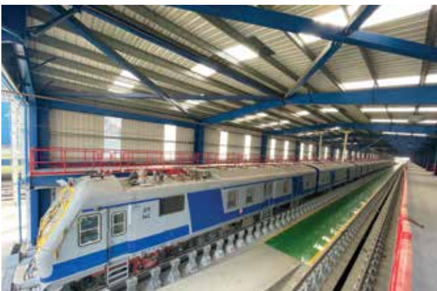
Railway MEMU Shed Woks, Kanpur, U.P
