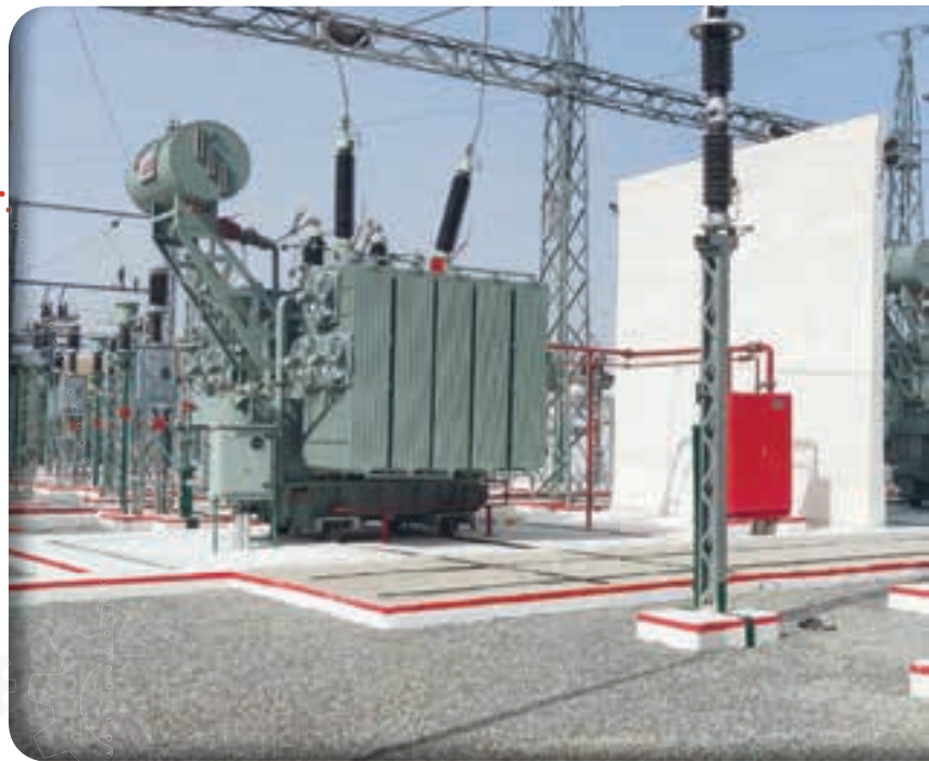
SS01 & SS04, 220/132 KVA Sub station works, Nagaland
