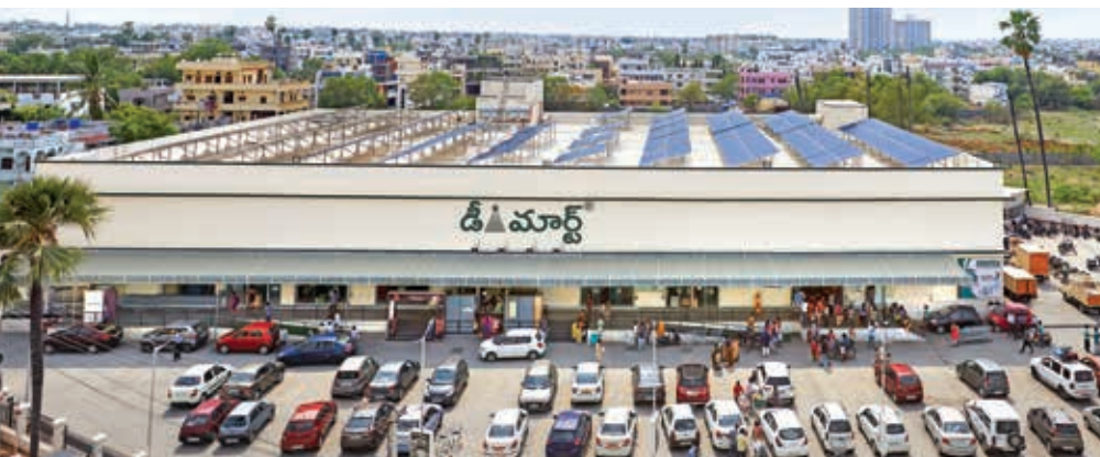
Rooftop Solar Panels
